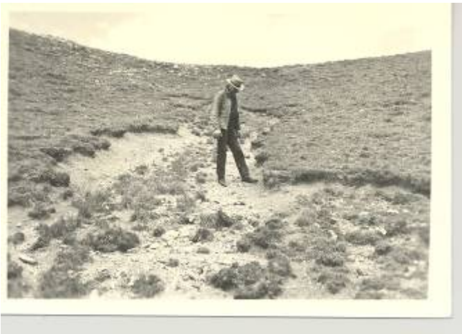
8/17/48. Early stages of erosion on sidehill near Ridge Driveway.
