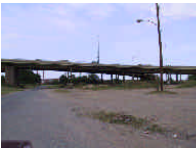
Bridge ramps at Poplar Point
