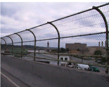
Pedestrian walkway on Frederick Douglass Bridge
