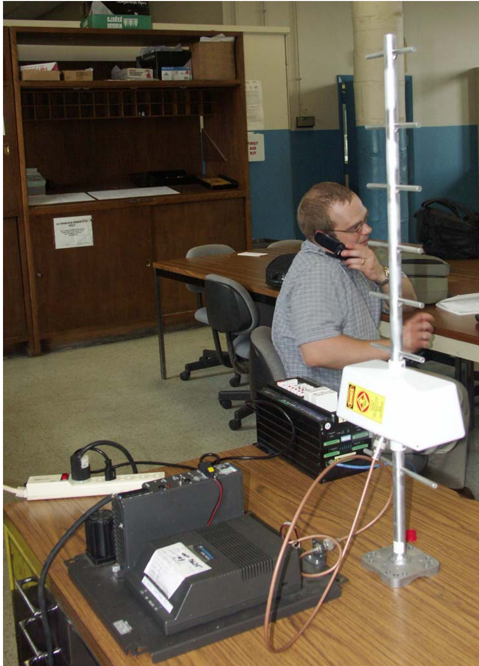
Figure 13. Radio and Antenna Used For Demonstration at Peoples Energy
