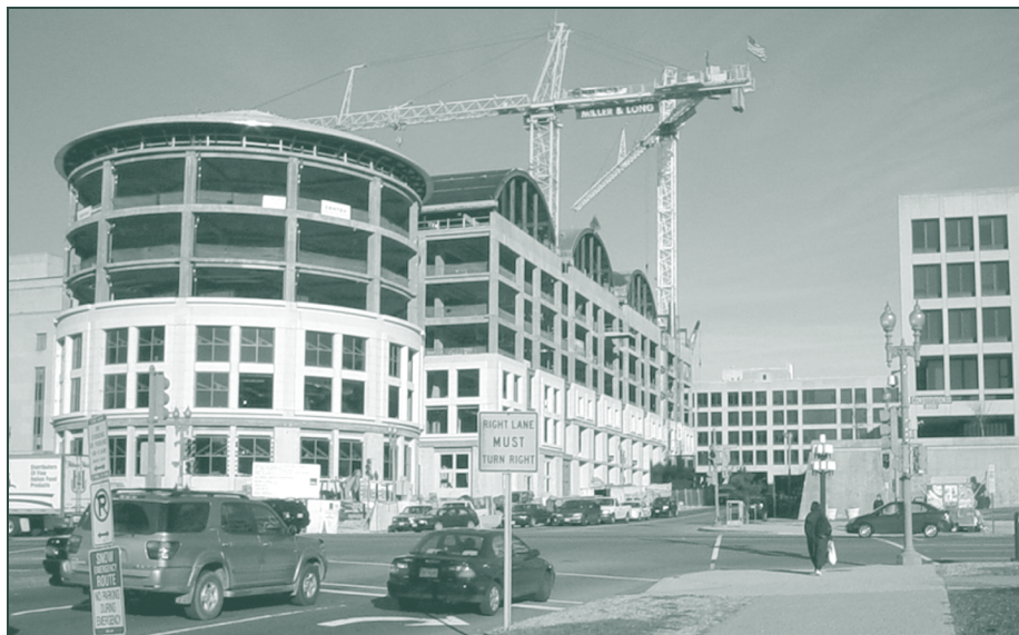
Construction of the E. Barrett Prettyman U.S. Courthouse Annex is underway.
