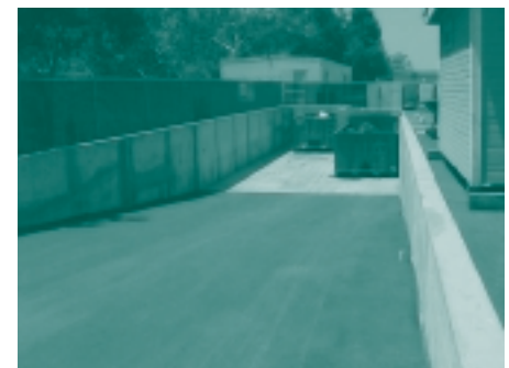
Side view of the paved ramp providing access for vehicles removing and replacing full roll-off containers.
