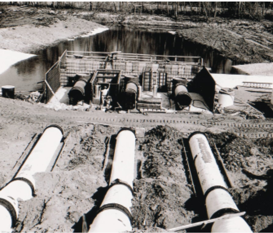
Figure 4-8. Levee districts combat groundwater seepage using drainage canal networks and large pumps like this one on the Sny Levee District in western Illinois (Source: St. Louis Post-Dispatch ).
