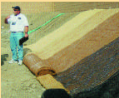
<Erosion-control mats for exposed landscapes (without vegetation) to prevent soil erosion, which is one component of runoff pollution>
