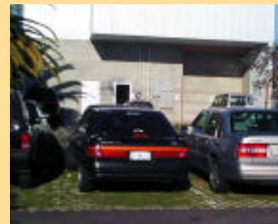
<Parking lot of small office building made of concrete permeable pavers>
