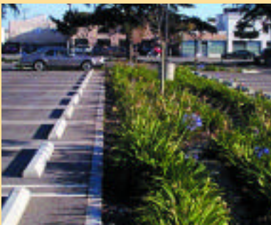
<Parking lot runoff enters biofilter for treatment and percolation, instead of flowing onto streets>
