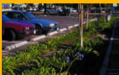
<Commercial parking lot biofilters>
