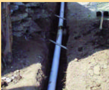
<Downspouts from roof gutters direct runoff into drywell>
