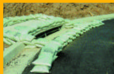
<Catch basin protection to reduce sediment loading>
