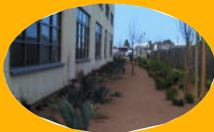
<Commercial biofilter sidewalks>
