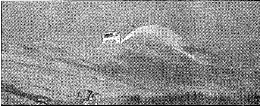
Figure 3-4. Soil Binder Application
