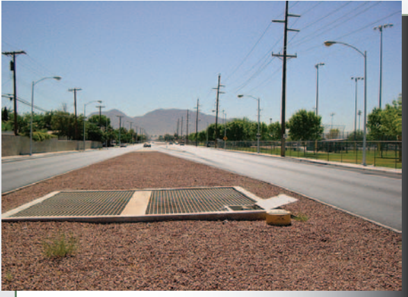
Las Vegas Creek at Lena Street (Washington Avenue Channel)
