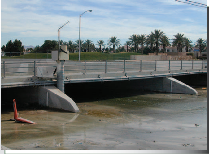
Flamingo Wash at Nellis Boulevard (Upstream of Las Vegas Wash Confluence)
