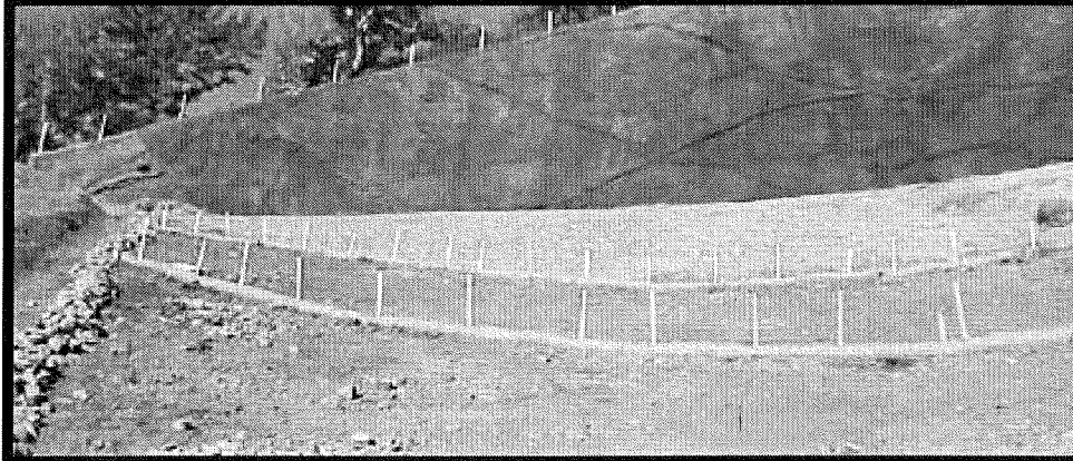
Figure 2-8. Benches and Retaining Wall on Slope
