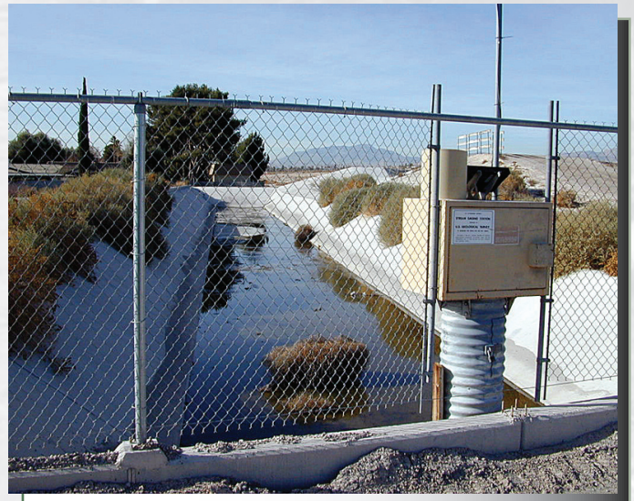
Meadows Detention Basin (at the Alta Channel)
