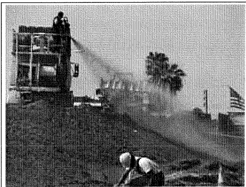
Figure 3-17. Hydraulic Mulch Application
