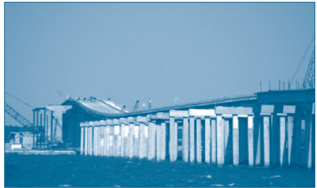
Newly built Bay St. Louis Bridge
