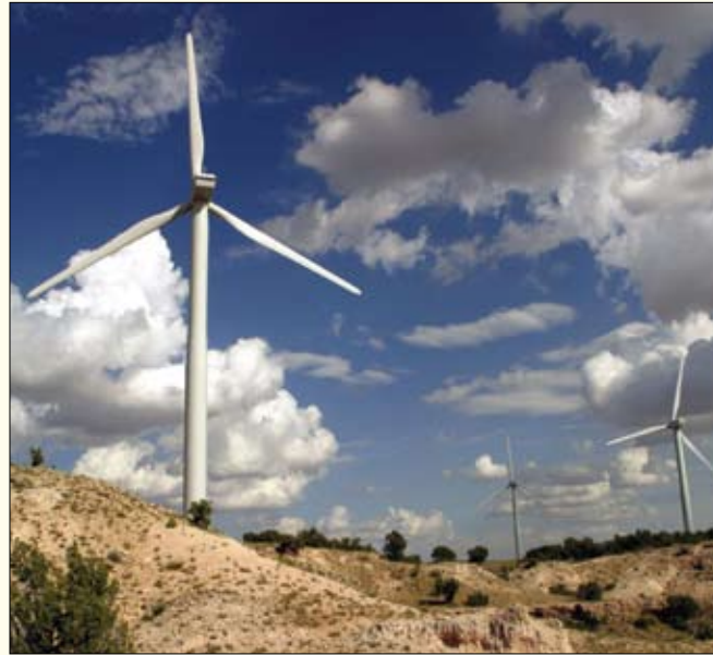
Turbines spin at the New Mexico Wind Energy Center, which recently started producing electricity for PNM. The center is the world's third-largest wind generation project.
