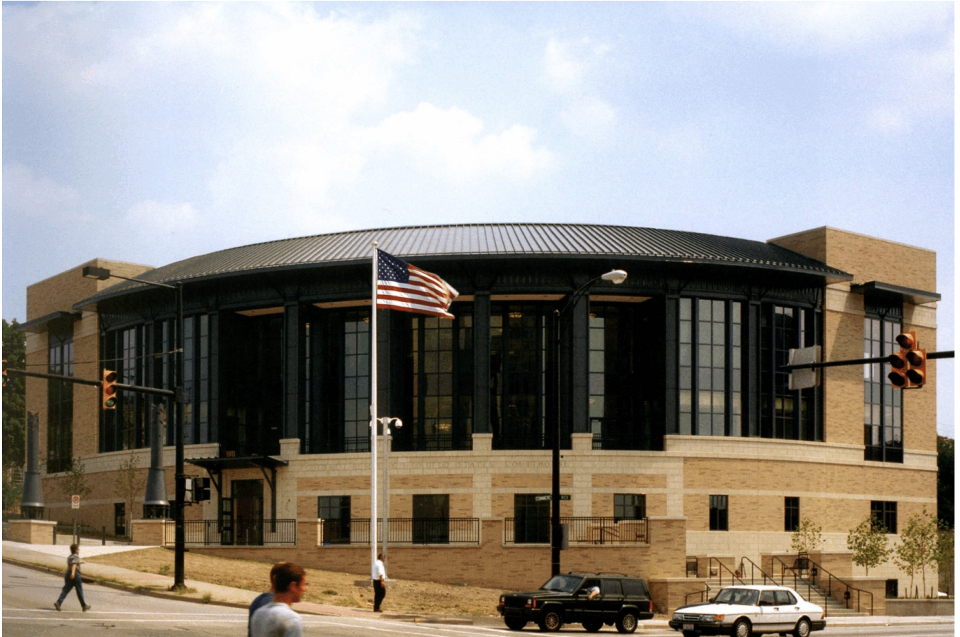
The Nathaniel R. Jones Federal Building and U.S. Courthouse Youngstown, Ohio
