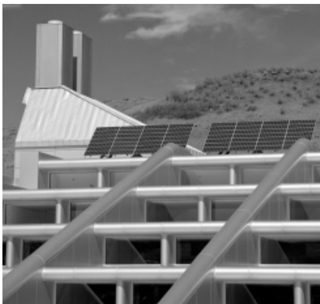
This energy-efficient laboratory building, built in Colorado in the 1990s, faces south and makes use of daylighting, evaporative cooling, and advanced heat recovery systems; the photovoltaic modules on the roof feed electricity into the local grid.
