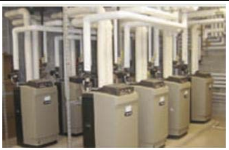
Modular Boiler installation: Courtesy of Weil McLain
