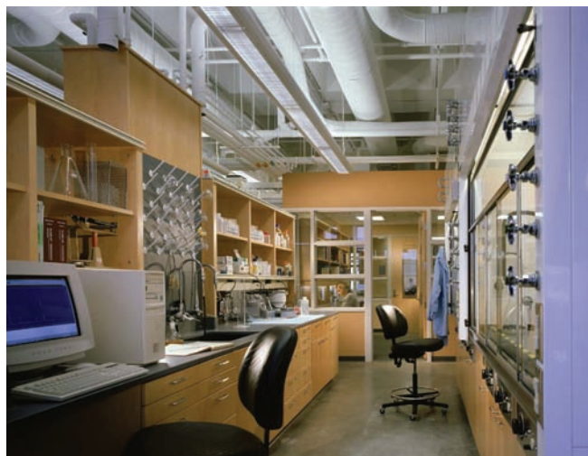
Figure 2: Left - Typical installation of direct-indirect lighting at the Donald Danforth Plant Science Center. Source: HOK. Right - Typical T8 direct/indirect lighting installation, University of Wisconsin Chemistry Building. This example shows that indirect lighting can be implemented even without a conventional ceiling. Source: Pivotal Lighting Design/Affiliated Engineers.
