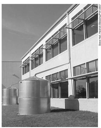
Figure 3. Exterior view of the Nidus Center shows the cisterns that store rainwater for irrigation and the exterior overhangs.
