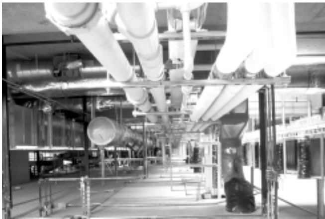
Interior view showing interstitial space.
