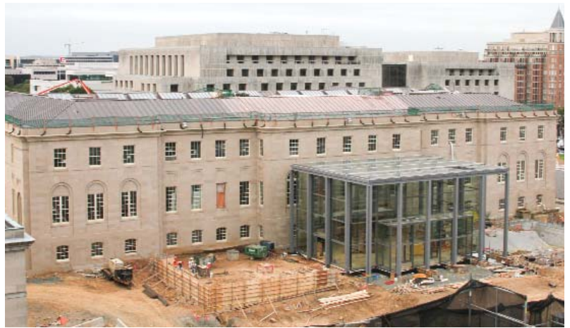
View of the D.C. Court of Appeals during modernization construction.
