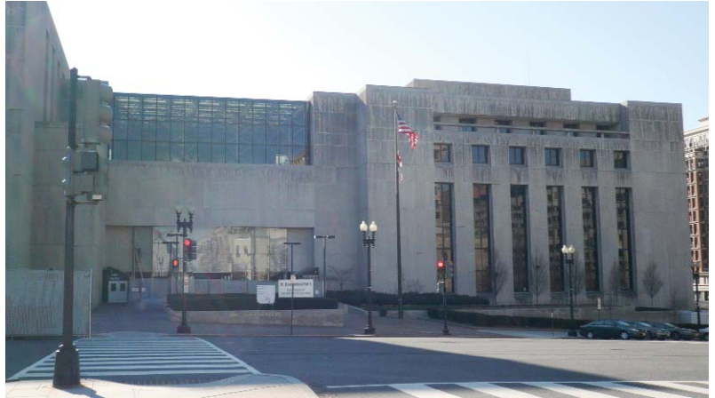
H. Carl Moultrie Courthouse undergoing improvements.
