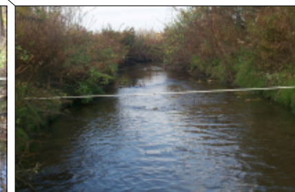
MIDDLE BRANCH OF CLINTON RIVER REACHE 20-22 DESCRIPTION: WIDE, SHALLOW RIVER, CONNECTED TO FLOODPLAIN RIVER TYPE: "E", BUT UNCHARACTERISTICALLY WIDE STABILITY: SLIGHTLY UNSTABLE (AGGRADATION) OTHER NOTES: SMALL CROSS SECTIONAL AREA COMPARED TO THE REST OF THE RIVER, GIVEN THE SIZE OF THE DRAINAGE AREA
