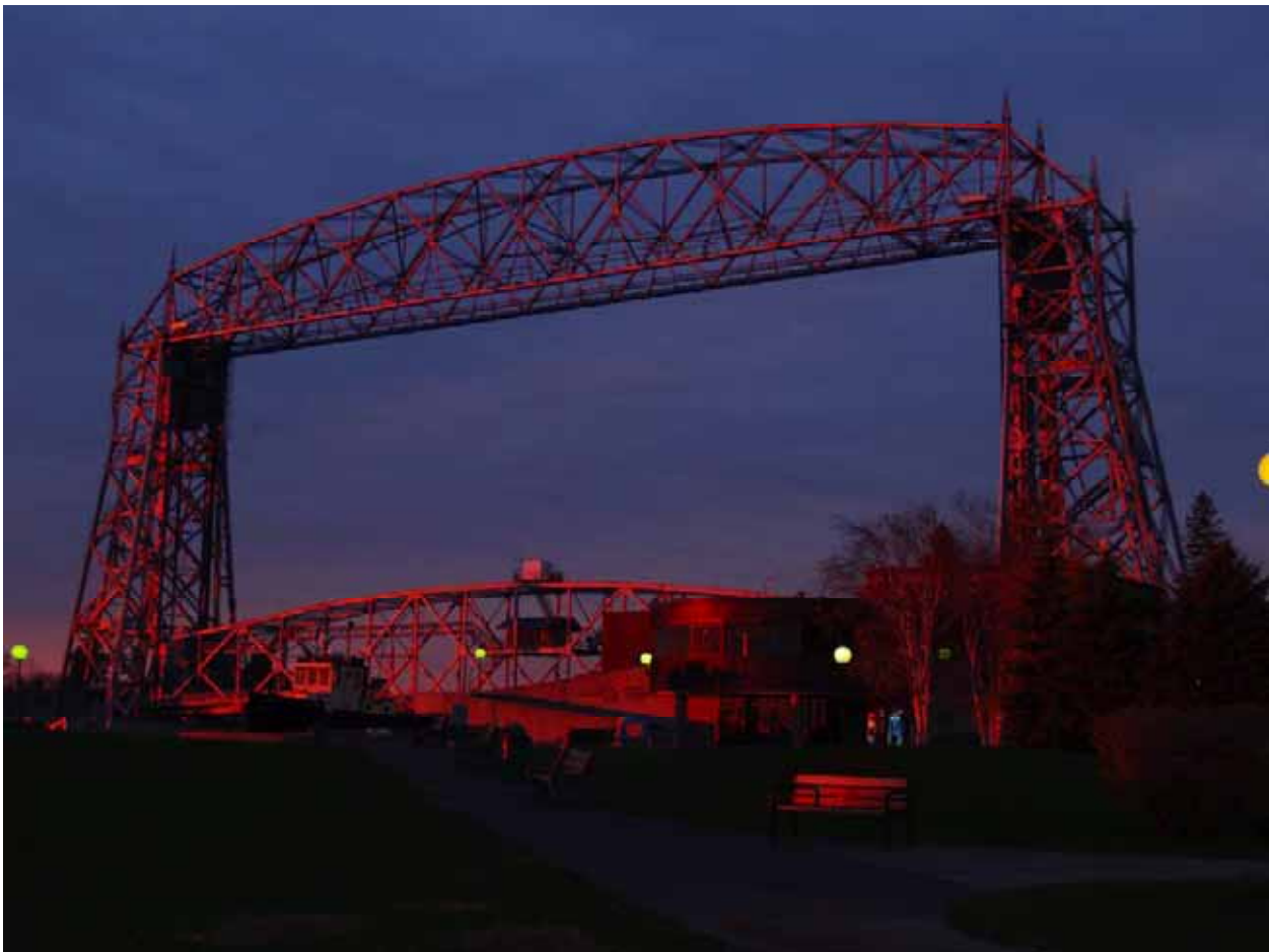
Figure 2. Duluth lift bridge early in the morning. Photo Credit: Cindi Kahrman, MPCA.
