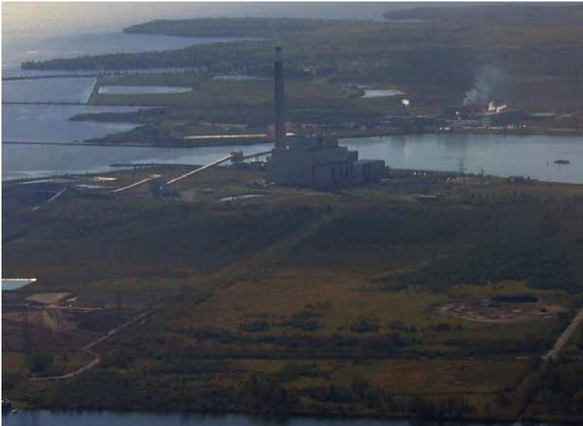
Ontario power generation facility, Thunder Bay, Ontario. Photo Credit: John Marsden, Environment Canada.
