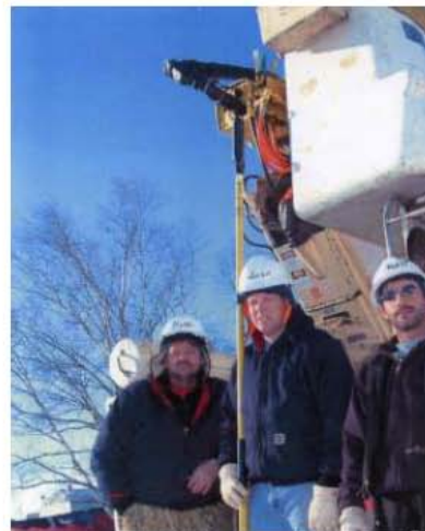
PCB transformer phase-out (Grand Marais, MN)
