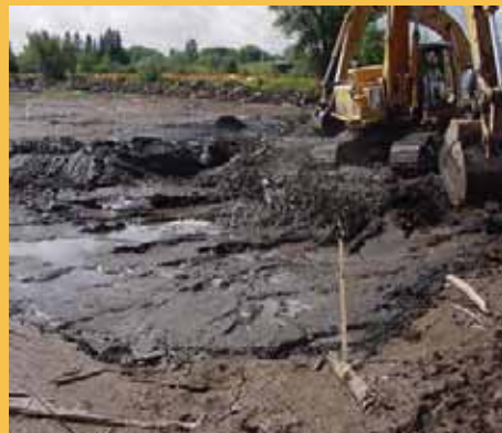
Contaminated sediment excavation at Hog Island, Superior, Wisconsin.
