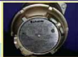
Non-mercury switch (left) used to replace a mercury switch at Murphy Oil Refinery.
