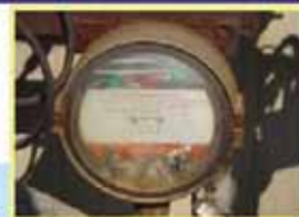
Non-mercury switch (left) used to replace a mercury switch at Murphy Oil Refinery.
