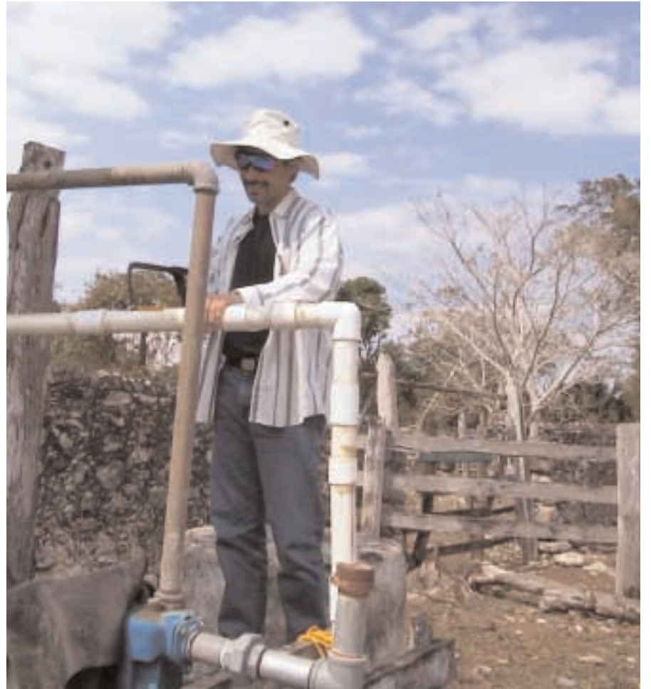
PV PUMPING— Sandian Michael Ross helps build a photovoltaic (PV) water-pumping station at a ranch near Cancun, Yucatan, Mexico.
