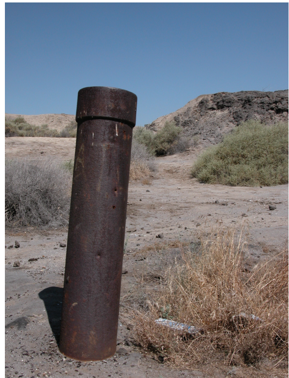
Figure 3.36. A closer view of the Lakewood 1 well casing as it appears today.
