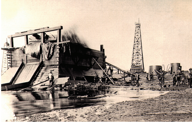
Figure 3.32. A box made of large timbers was pulled over the Lakeview gusher with cables. Photograph courtesy of Don Arnot, West Kern Oil Museum.
