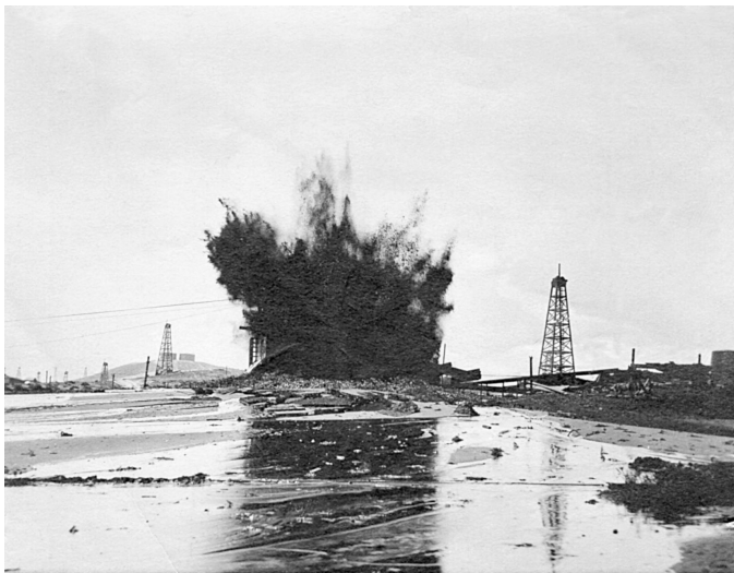
Figure 3.33. The box was not able to contain the force of the gusher. Photograph courtesy of Don Arnot, West Kern Oil Museum.
