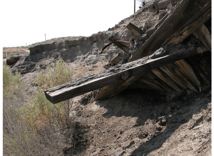
Figure 3.39. Remains of the embankment built to contain the Lakeview gusher.
