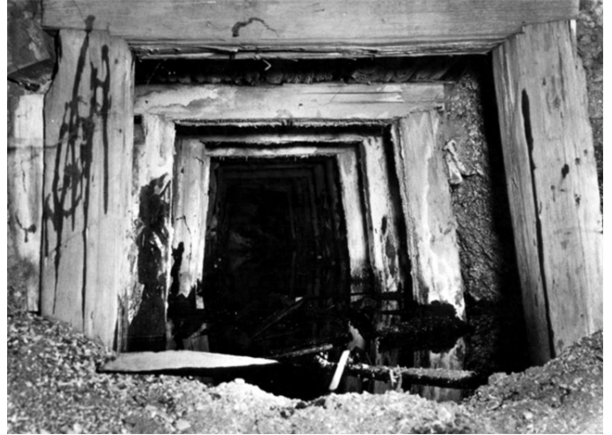
Figure 3.9. This mineshaft in the McKittrick asphalt mine, Kern County, was built in the 1860s with redwood timbers. Photograph by W. Rintoul, from Onshore Oil and Gas Seeps in California ( http://seeps.wr.usgs.gov/seeps/index.html ).
