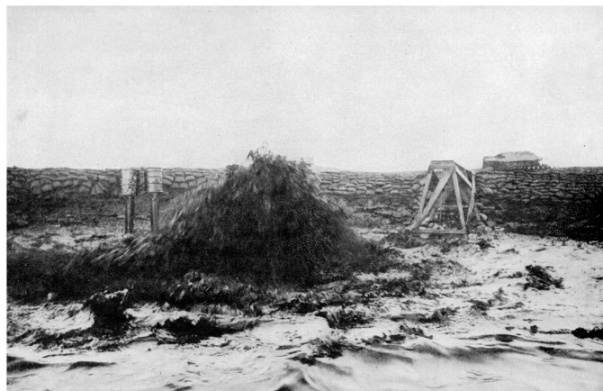
Figure 3.34. A dam of sandbags was built around the Lakeview 1 well. This photograph was taken on October 2, 1910. Photograph by W.C. Mendenhall in Pack (1920).
