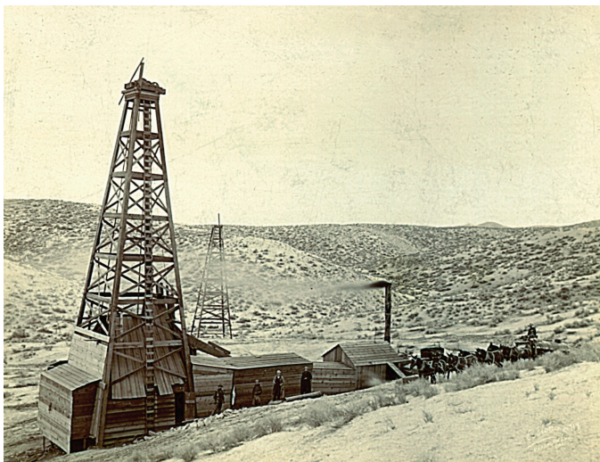
Figure 3.19. Wooden derrick and sheds housing the steam drilling rig. Photograph courtesy of Don Arnot, West Kern Oil Museum.
