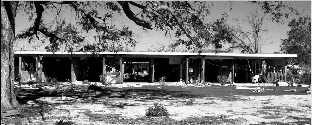
Figure 1. Photo of Destroyed Selected Nursing Home in Mississippi
