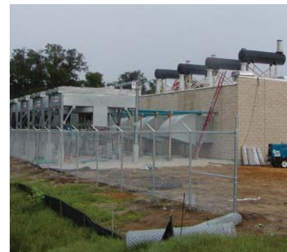
Landfill Gas to Energy Construction Geneva, FL
