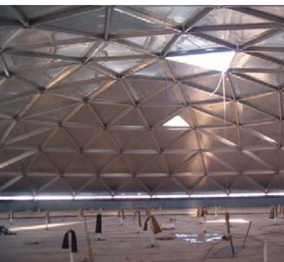
Geodesic Dome Construction Long Beach, Colton, CA
