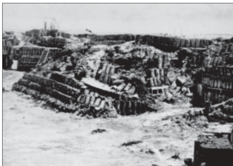
Figure 2.7: As artillery barrages reduced its masonry surfaces to rubble, Fort Sumter was revetted with gabions filled with cotton and sand - effectively making it into an earthen fortification - and more resistant to attack. Library of Congress.
