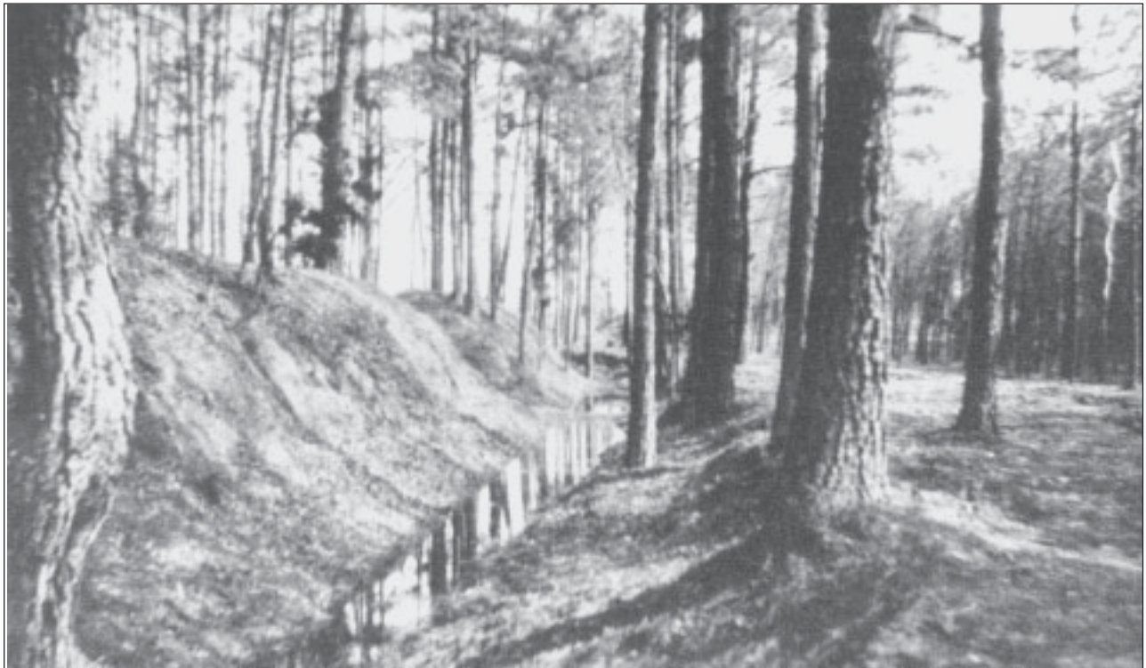
Figure 2.53: This view of Fort Welch's eastern parapet clearly shows the fish Hook access road to the right, mid-succession pines and hardwoods with a cleared understory immediately surrounding the historic fortifications. The back of the original photo is given the caption, 'clearing complete.' Petersburg NB archives.
