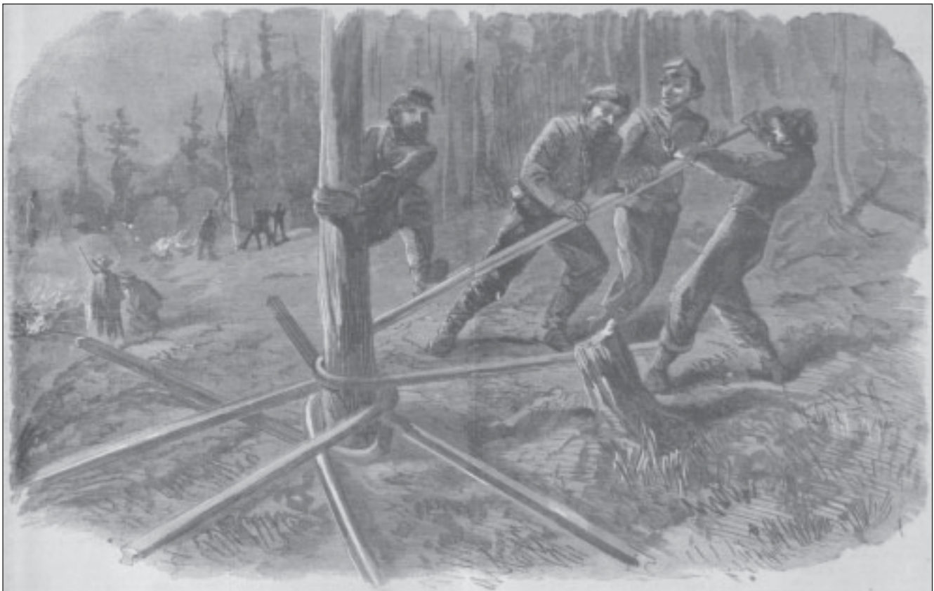
Figure 2.10: Federal troops heated captured southern rails over fires fueled by cross-ties, then bent them into forms popularly known as 'Grant's hairpins.' Harper's Weekly 31 December 1864.
