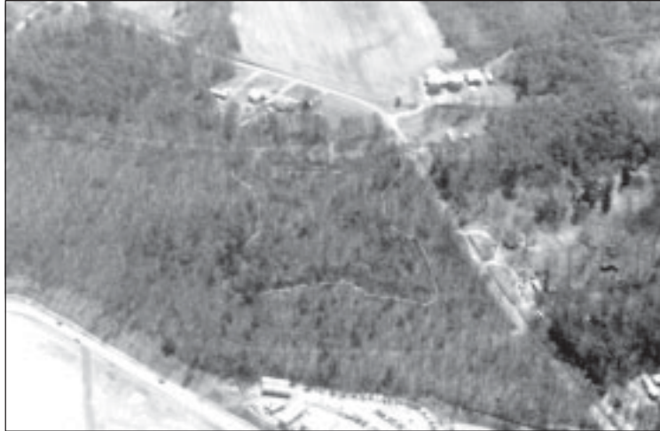
Figure 3.15: Oblique aerial photograph of Fort Fisher from the north, looking south. This view establishes a context for Fort Fisher's current setting, amidst blocks of woodland, bordered by Flank Road to the south and Church Road to the west. The cleared land of the steel recycling plant is seen in the foreground to the left. A light grey line has been added to this graphic to aid in visibility of the fort. Photo by the author.
