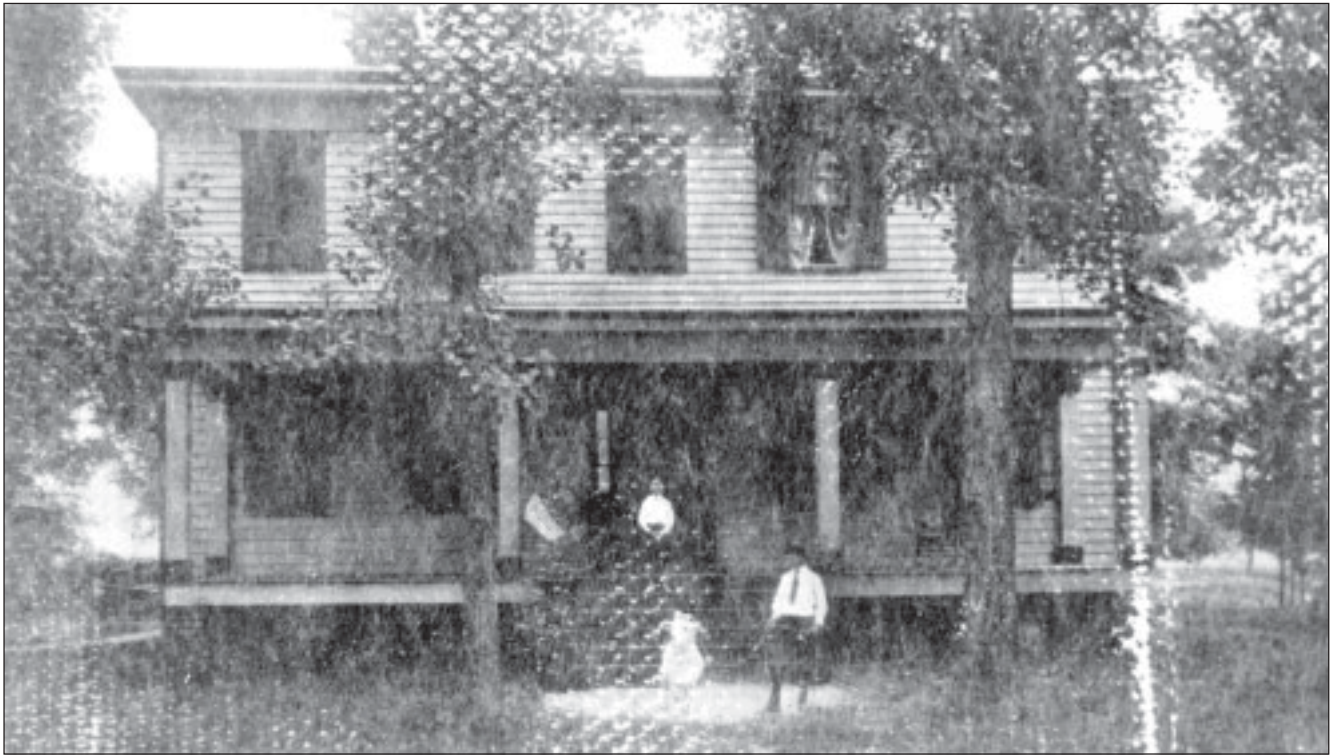
Figure 2.45: This dwelling, named 'Fort Fisher Farm' was built from timbers salvaged from the Federal signal tower by William Lemuel Peebles. The scale of the square porch supports is similar to the dimensions of the timbers used on the tower. Note the billygoat on the front walk. University of Virginia Special Collections.
