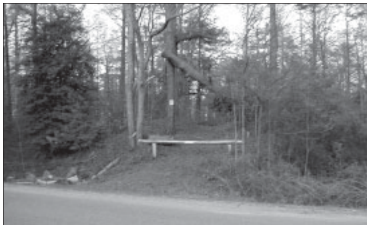
Figure 3.18: This view of Fort Fisher's southwest bastion shows the original ditch filled with soil to create a ramp for park maintenance vehicles. Photo by the author.
