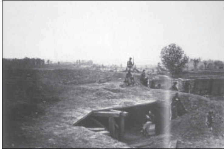
Figure 2.17: Bombproofs built of logs and soil protected soldiers from artillery blasts, flying shrapnel, exploding shells and inclement weather. Library of Congress.
