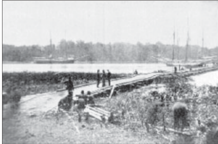
Figure 2.13: This pontoon bridge carried the Army of the Potomac towards Petersburg in June of 1864. Patriot Publishing Company.
