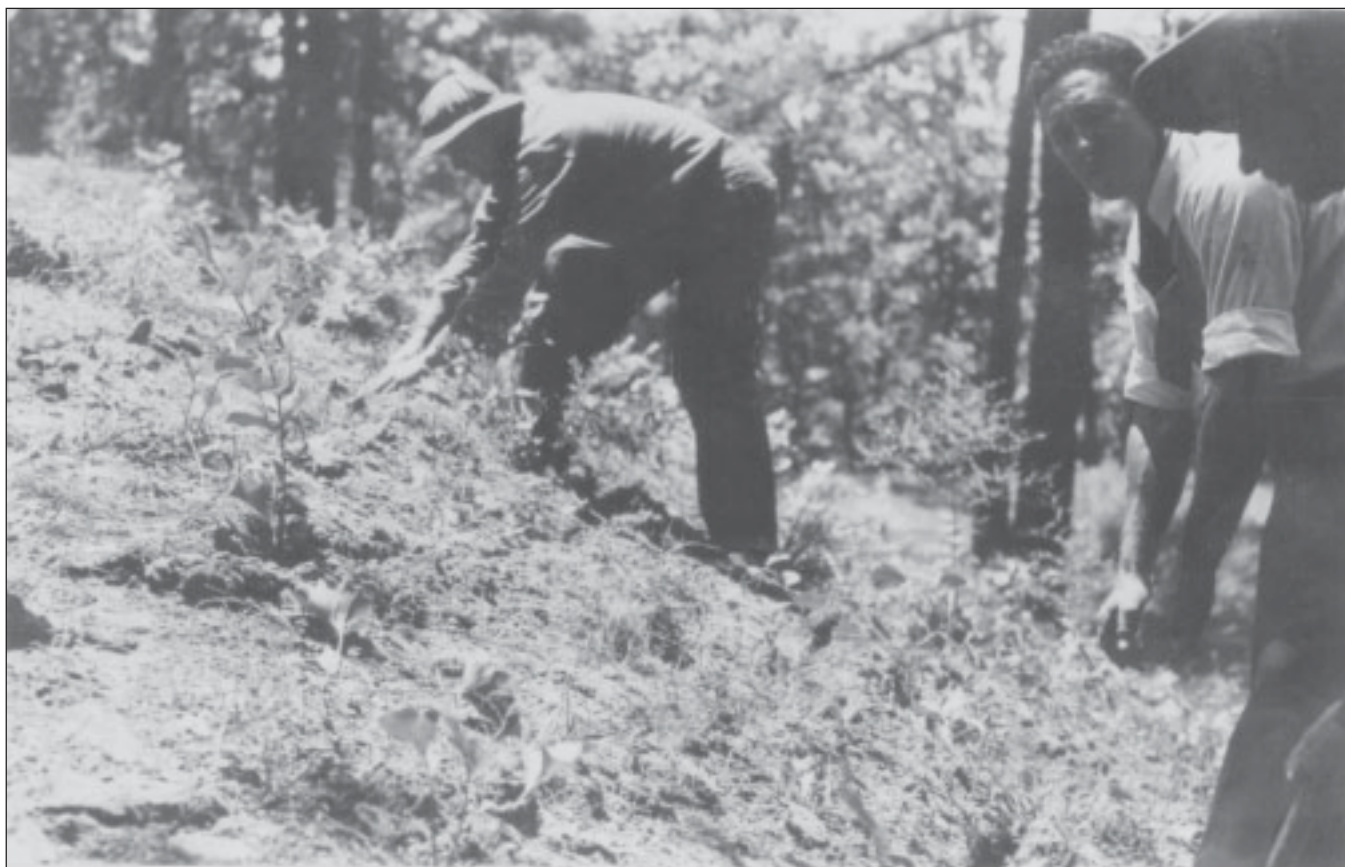
Figure 2.51: This photograph taken during April of 1934, shows CCC members ‘plugging’ Bermudagrass into the parapets of Fort Welch. In addition to the Bermudagrass, it appears that small shrubs have been planted on the berm. Note the mid-succession pines in the background. Petersburg NB archives.
