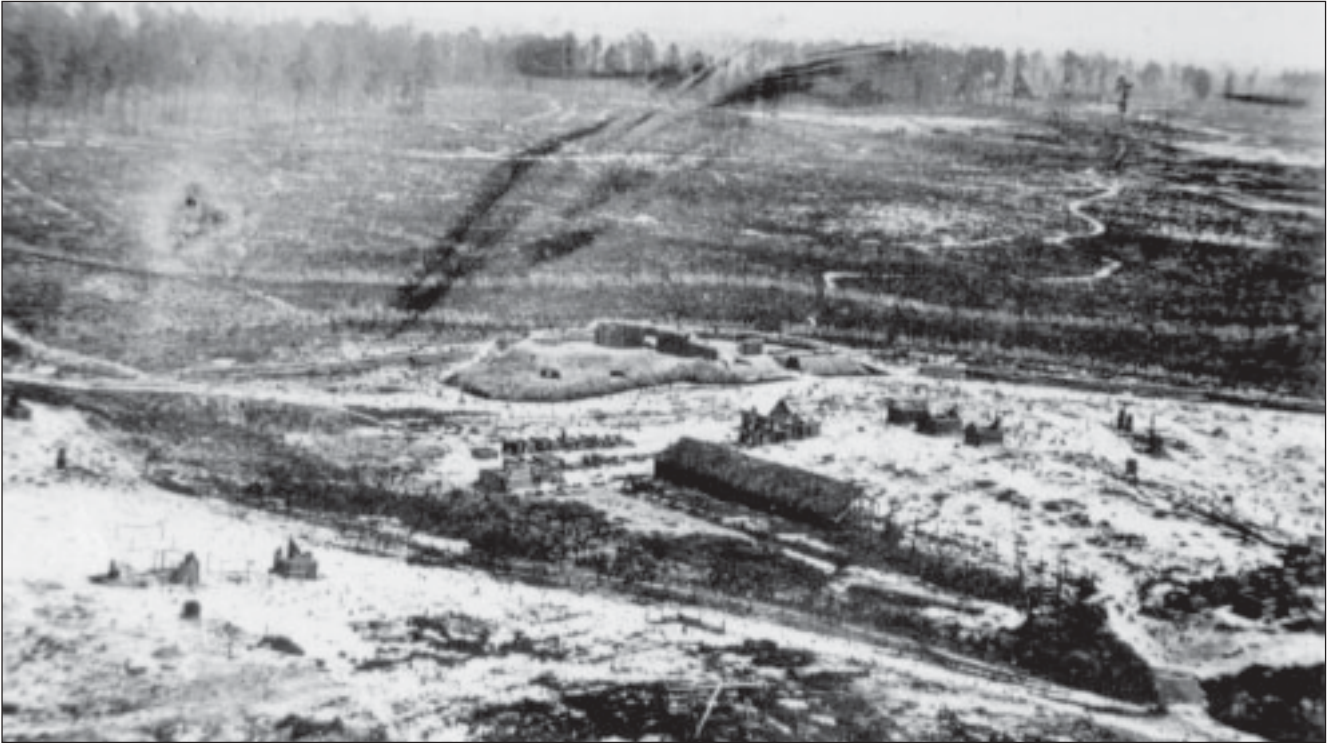
Figure 2.37: This photograph taken from the Union Signal Corps' tower at Peebles' farm, clearly documents the heavily slashed woodland north of the Federal Left Flank. Notice the casemate openings for artillery built into the fort, which was unusual for an earthen fort. Also evident is the log palisade which served as a traverse dividing the fort. Library of Congress.
