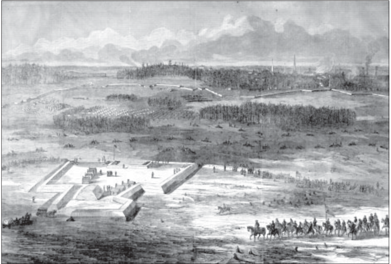
Figure 2.36: This engraving, probably made from a photograph taken in early 1865 from the nearby signal tower on Peeble's farm, shows work underway on Fort Fisher's expansion into a four-bastioned fort - the largest fort constructed on the Union siegelines surrounding Petersburg. The Confederate camps, the Southside Railroad and Petersburg's steeples are visible in the distance. Library of Congress.
