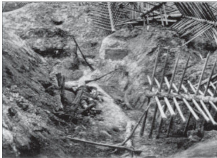
Figure 2.6: Rows of sharpened stakes placed out in front of fortification were used to help repel an attacking force. Library of Congress.
