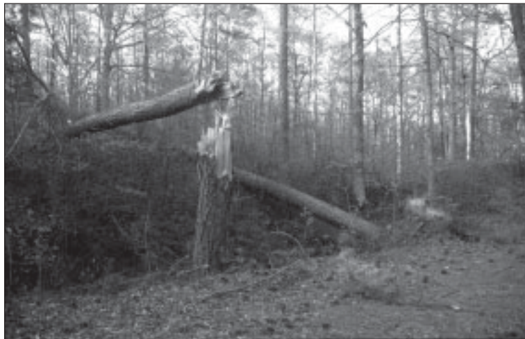
Figure 3.4: Storm induced blow-down of large caliper trees such as this on the parapets of Fort Fisher create a potentially dangerous condition for visitors and work to destroy the physical integrity of the historic earthworks. Photo by author.
