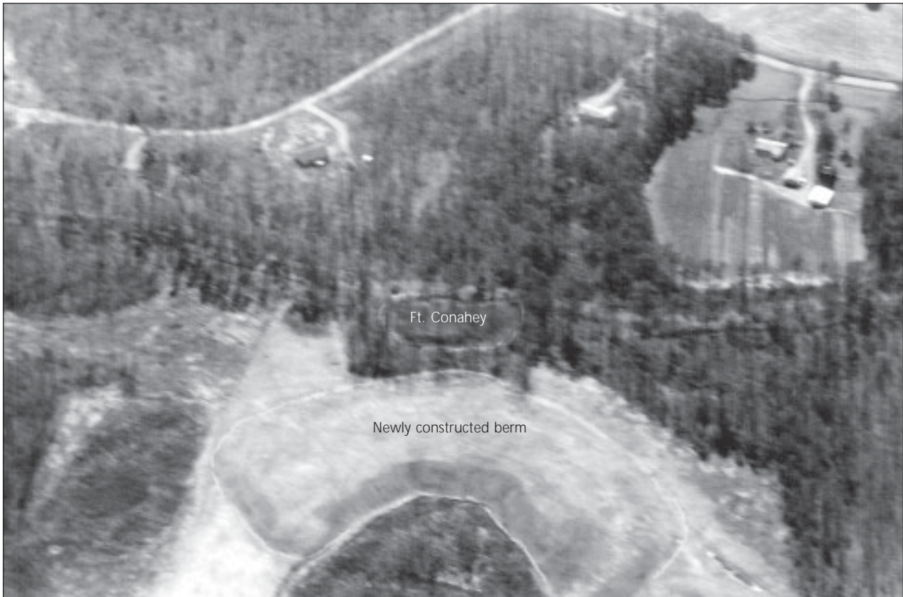
Figure 3.7: This aerial view of Fort Conahey shows its proximity and scale compared to the oversized earthen berm installed by the steel recycling plant. The berm was intended to block the steel plant from view. Fort Conahey and the berm have been outlined with a light grey line for visibility. Photo by the author.
