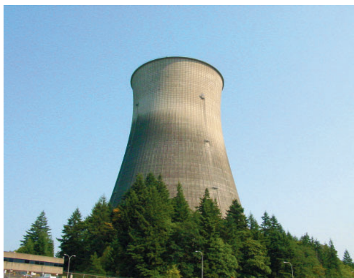
Figure 9: Trojan cooling tower The Trojan Nuclear Power Plant cooling tower was imploded in May 2006 as part of the plant's decommissioning.
