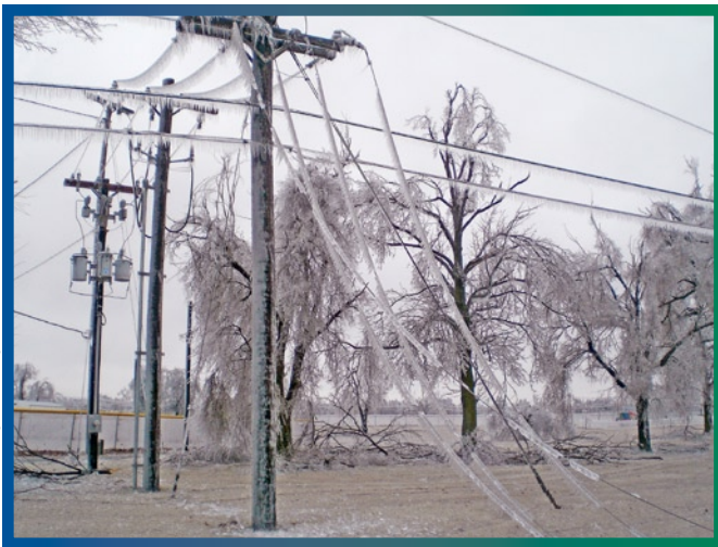
LOCAL DISTRIBUTION LINES IN AND AROUND KENNETT, MISSOURI, WERE TORN DOWN BY THOUSANDS OF POUNDS OF ICE.
