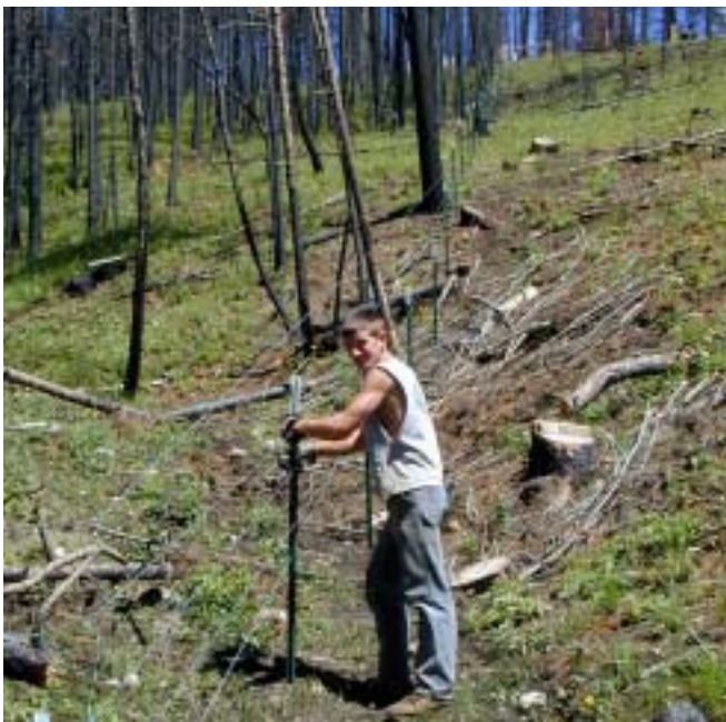
Replacing fences destroyed by wildland fires on private lands in ID.
