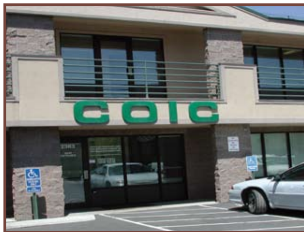
Central Oregon Intergovernmental Council headquarters, Redmond, Oregon.
