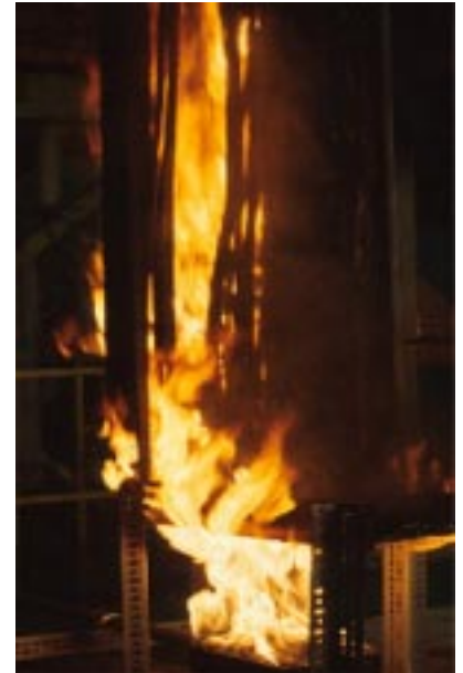
Figure 8. Fire spread through a cable bundle mounted vertically.
