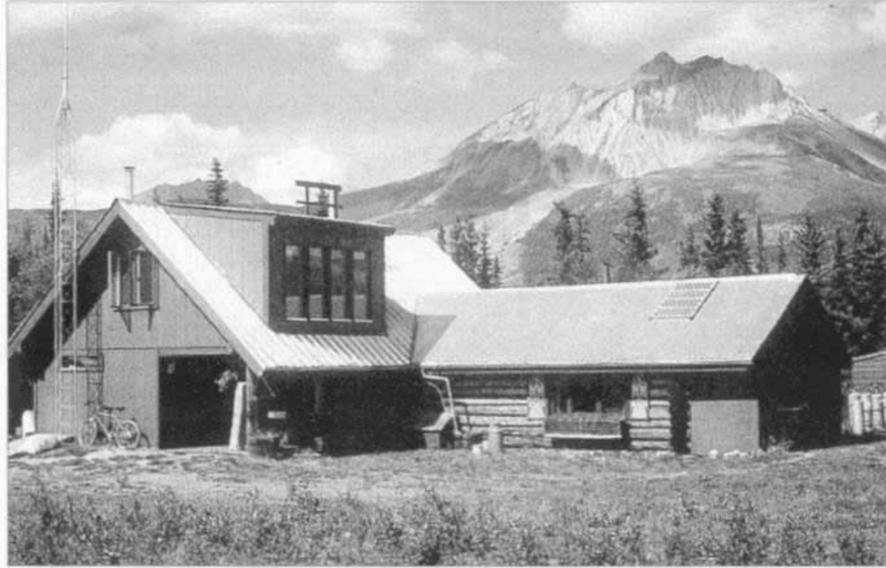
May Creek Operations Center
