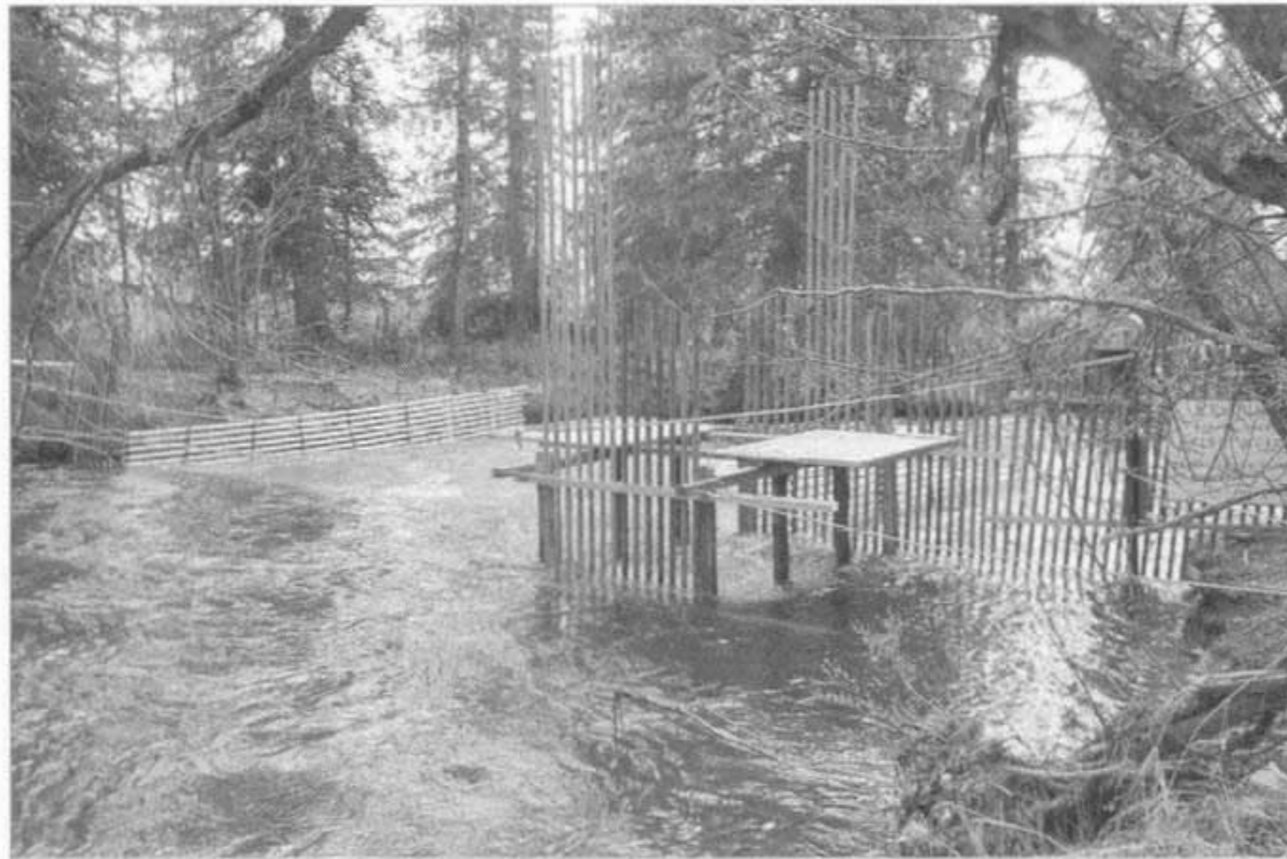
In 2001 WRST installed a newly-designed floating weir in Tanada Creek
