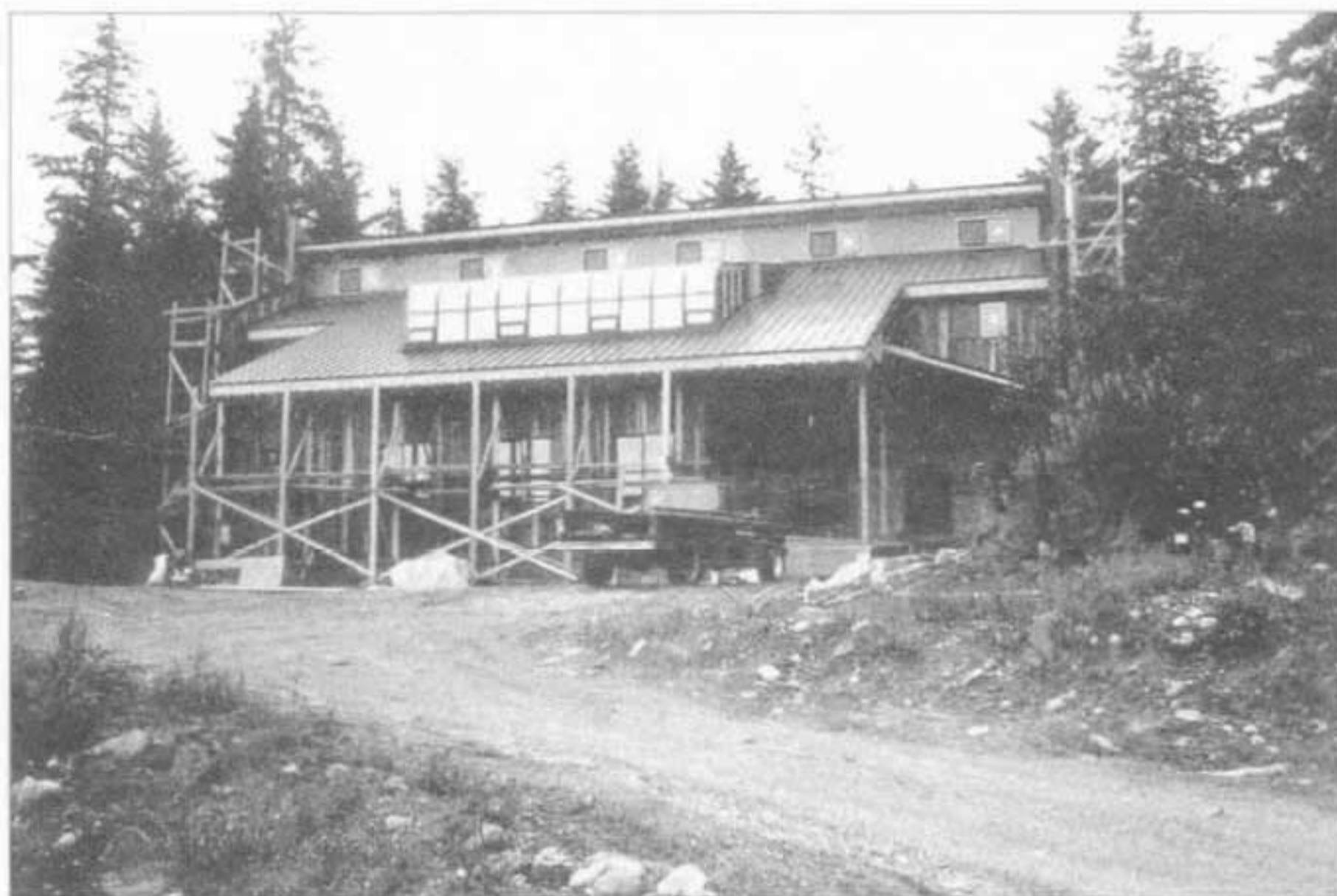
WRST's current Yakutat facility was constructed in 1993
