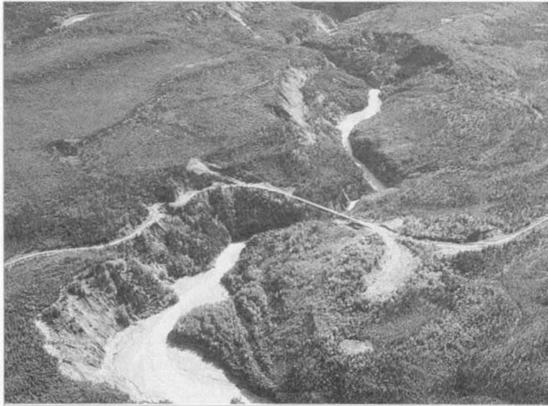
Aerial view of McCarthy Road, showing Kuskulana River Bridge
