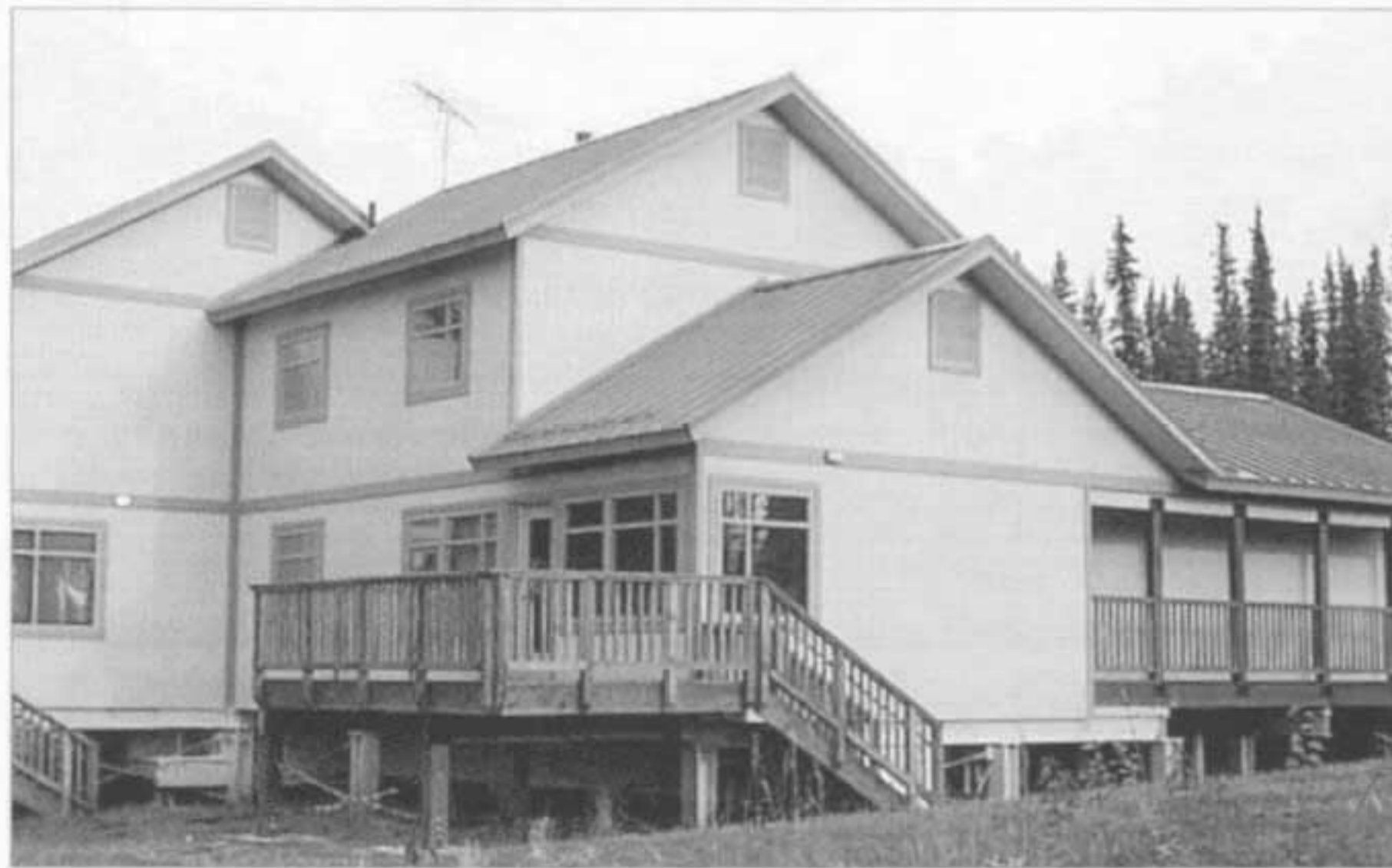
WRST and the BLM share this modern housing facility in Glennallen
