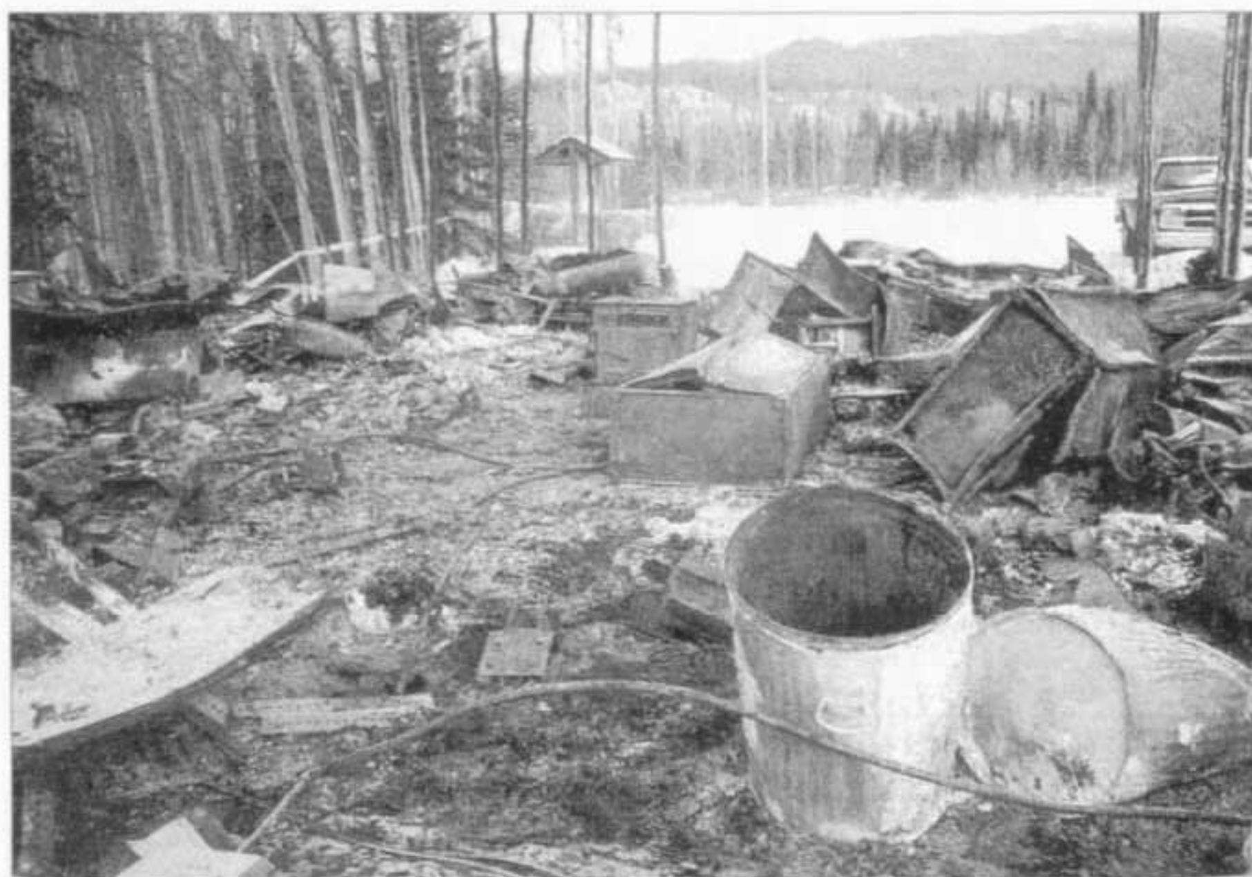
The Slana Ranger Station following the 1992 fire
