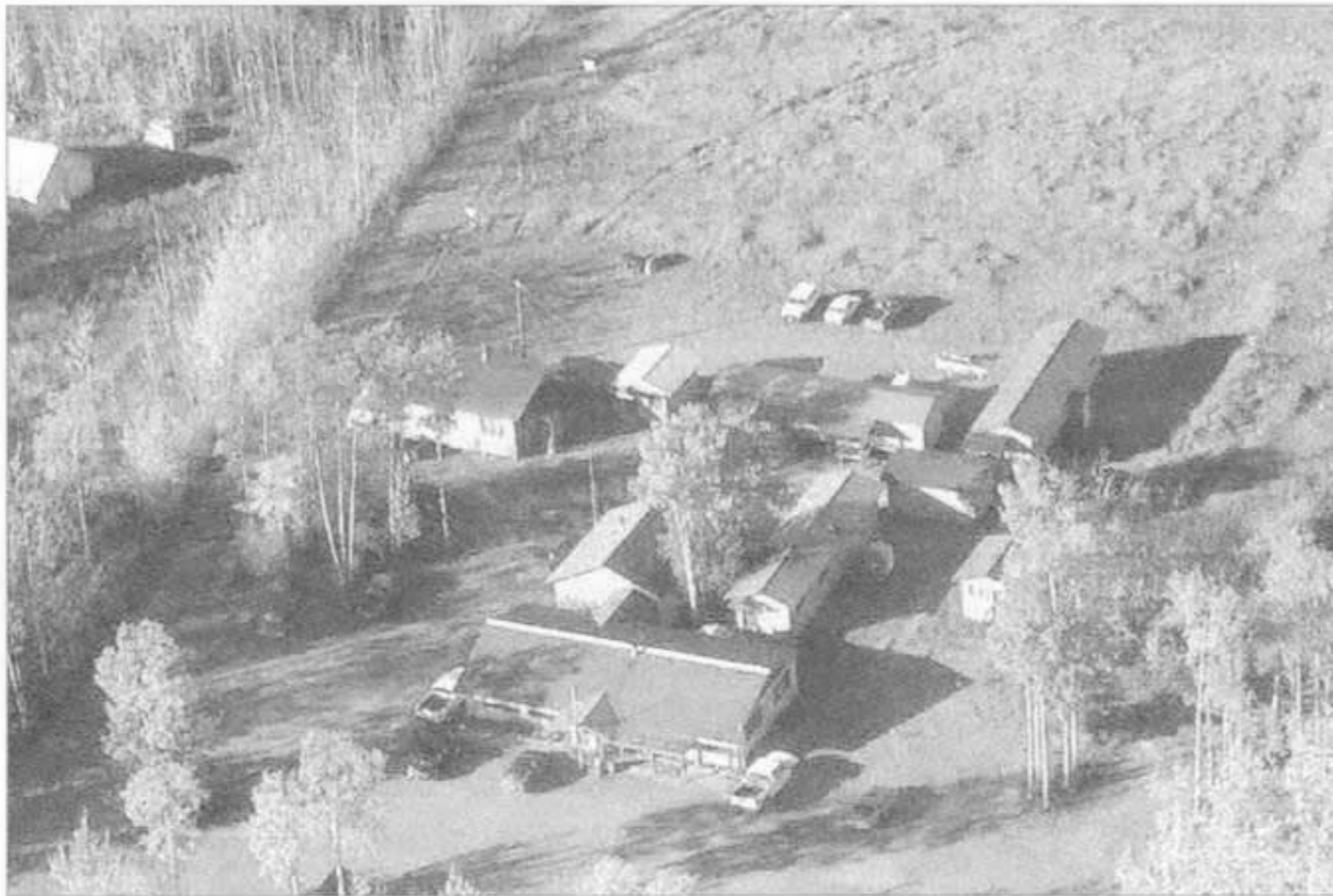
WRST's headquarters complex in Copper Center
