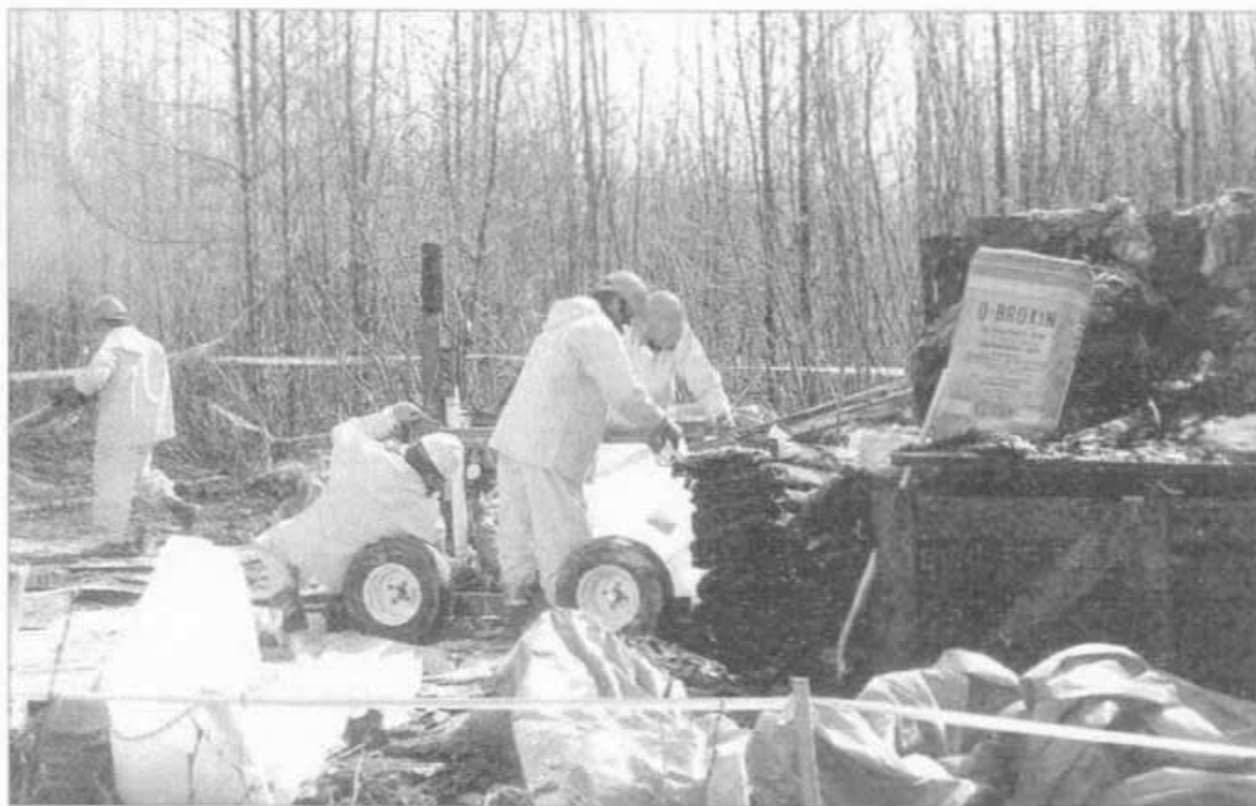
Crews removing hazardous materials at Sudden Stream
