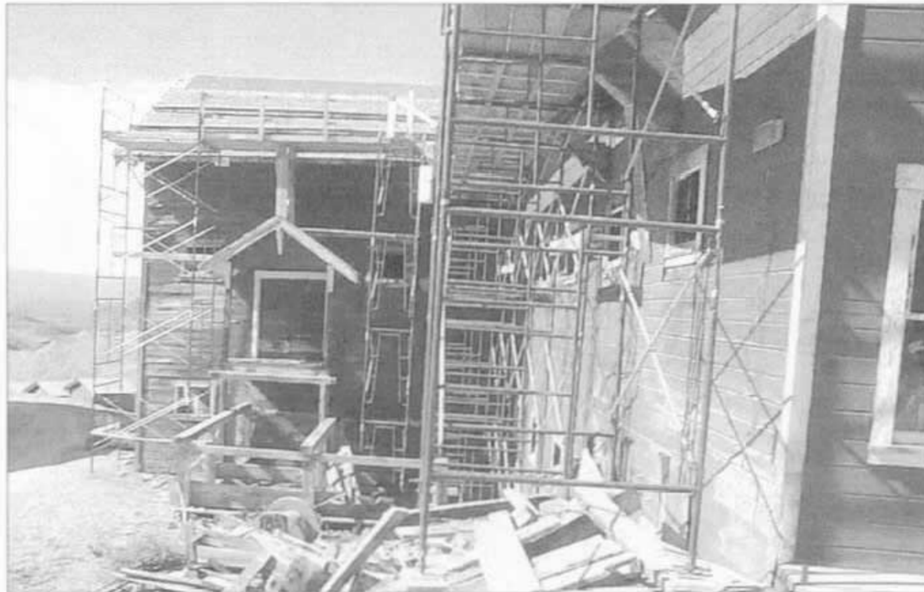
WRST began its stabilization efforts at Kennecott in 1999
