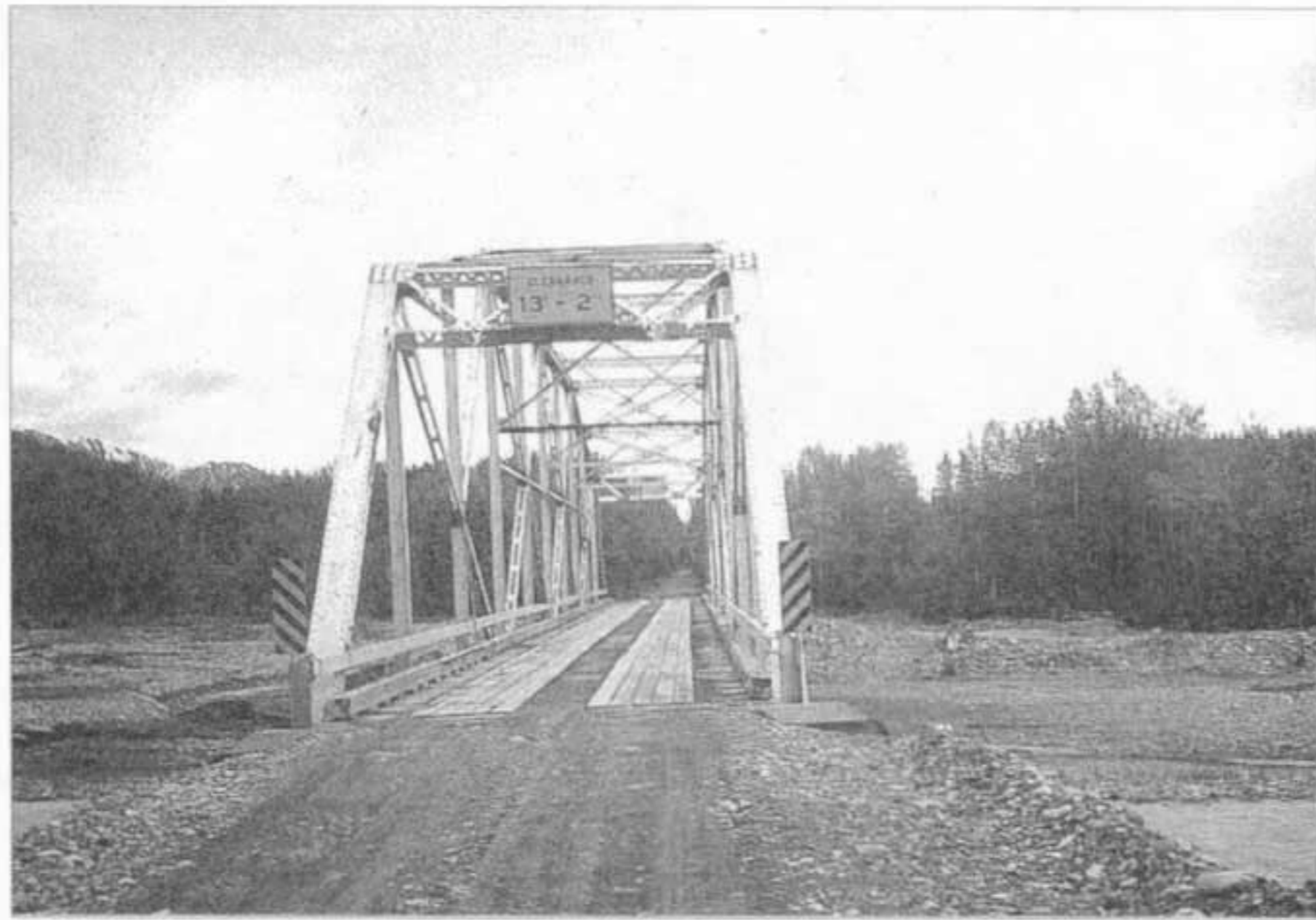
Recycled one-lane bridge over the Lakina River
