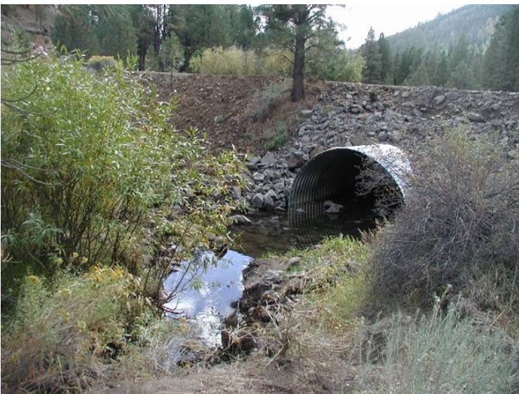
Dog Creek Culvert Replacement Silver Lake Ranger District
