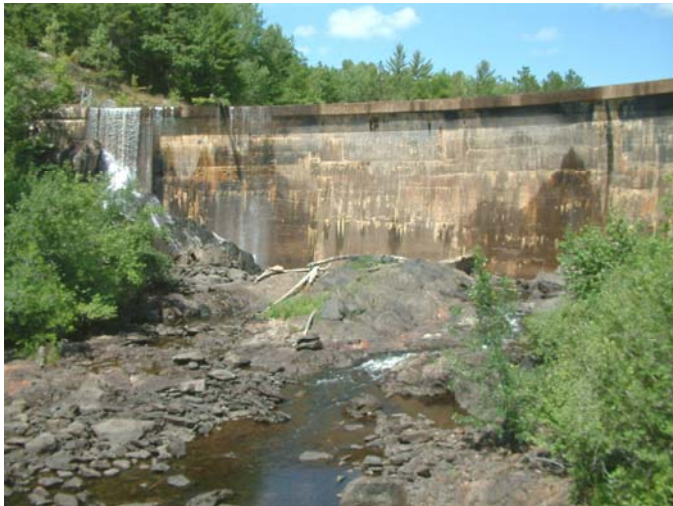
The dam site before removal
