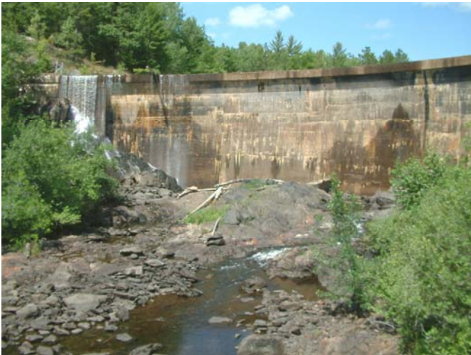
The dam site before removal
