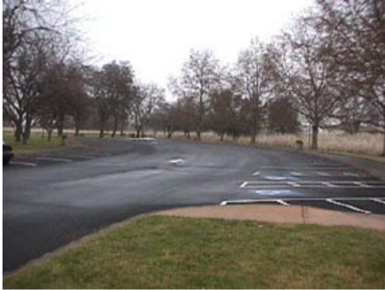
The main parking lot next to the visitor center will be reconfigured to make more efficient use of the space and to allow for bus and RV parking
