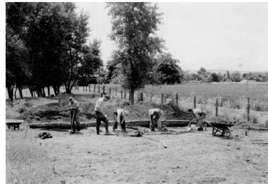
Excavation of Mission House 1941
