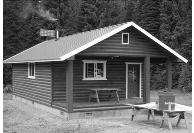
The new Roundtop Trail Shelter.
