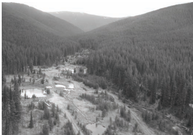
Excavation of the flood plain. Photo Lisa Hawdon
