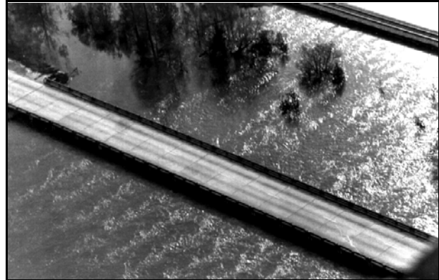
Figure 1-3. A highway bridge that creates complex hydraulic conditions by constricting floodplain flows at high stages.
