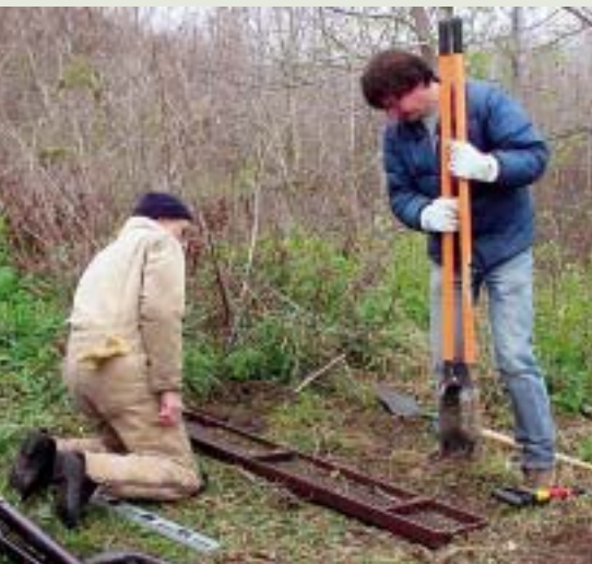
Arrow Rock Mayor Tom Beamer calls the trail “a bonus for the town,” a historic community that saw the Missouri River move away from the town limits as floods cut the link. Friends of Big Muddy Volunteers Peter Ironwood, left, and Troy Gordon installed a bench along the trail as construction moved forward in November 2003. (Janine Gordon)
