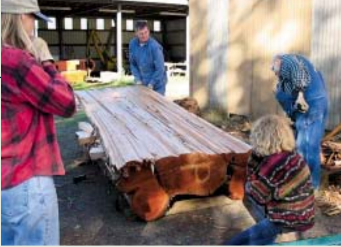
The Cathlapotle Plankhouse will cost approximately $500,000 to build. More than 50 volunteers have put in more than 2,000 hours so far building a 78-foot-long plankhouse that recreates the economic and residential centers of Chinookan households. Volunteers Ginger May (left), Larry Siewert (center; rear), Tom Laidlaw and Becky Railey used wooden wedges and lots of trial and error to split a 3-inch-thick plank from a donated cedar log. (Virginia Parks/USFWS)
