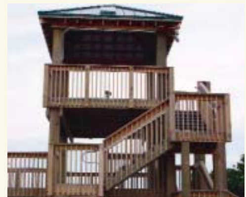
J.N. “Ding” Darling NWR, FL, used fee monies to build an observation tower, redesigned to help comply with the Americans with Disabilities Act. The main level platform was expanded and an ADA-compliant ramp was installed. The refuge also completed rehabilitation on the Indigo Trail, installing a boardwalk with recycled plastic lumber and two rest benches. (USFWS)
