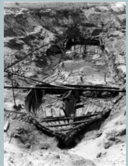
With excavation about half completed in 1969, the forward part of the Bertrand had been made visible and the mud had been cleared. The decking over the midsection was still in place. Cargo can be seen in the boat's hold below the edge of decking. The Bertrand sank April 1, 1865, after hitting a snag in the Missouri River on its way to the gold fields of Montana. (Photo by Leland A. Larson, courtesy of Woodmen of the World magazine)
