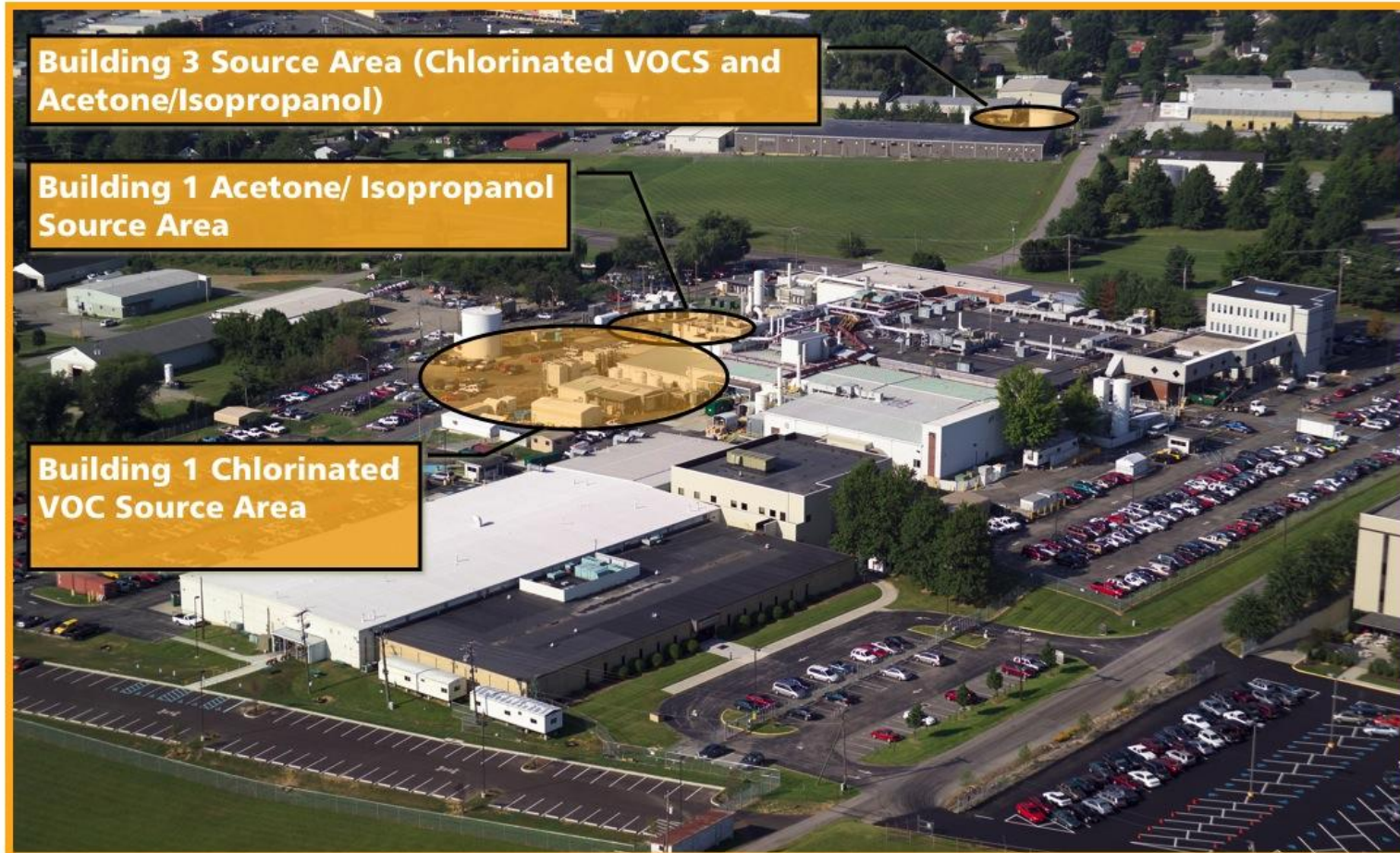
Figure 2. Photograph Showing Source Areas
