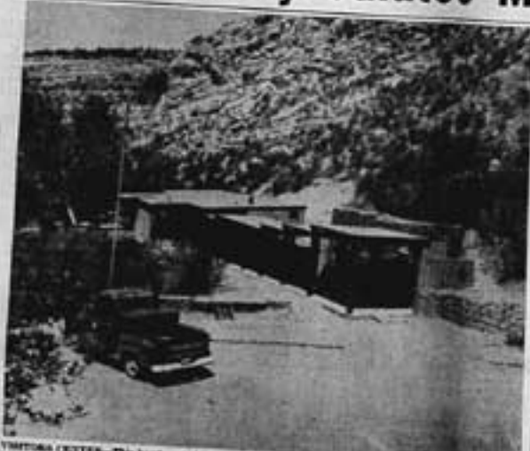
VISITOR CENTER —This handsome structure was built at Montezuma Castle National Monument...
