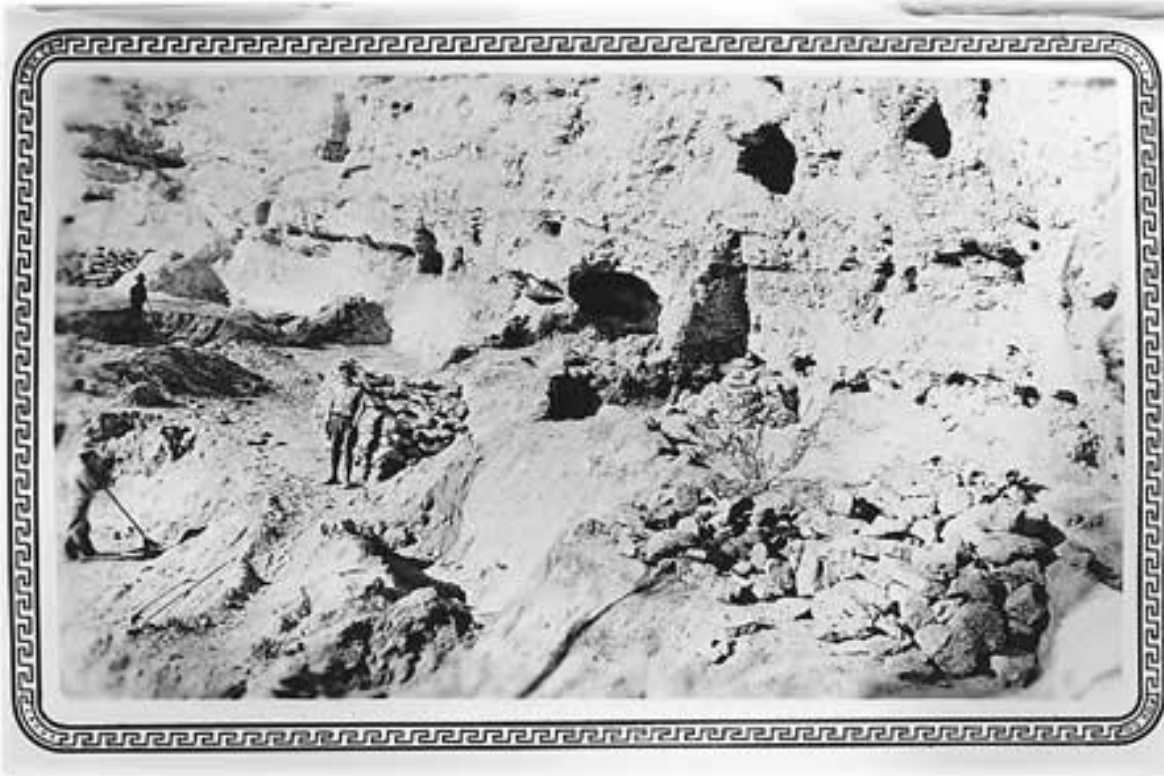
Figure 20. Castle A from the east, after the second tier of rooms was cleaned. From the report by Martin L. Jackson entitled, "Report on Montezuma Castle C.W.A. Work, Federal Project No. 5," National Archives, Record Group 79, box 2289, folder 619 (Civil Works).
