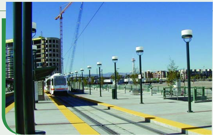
Light rail system behind Denver Union Station, with new commercial development in the background
