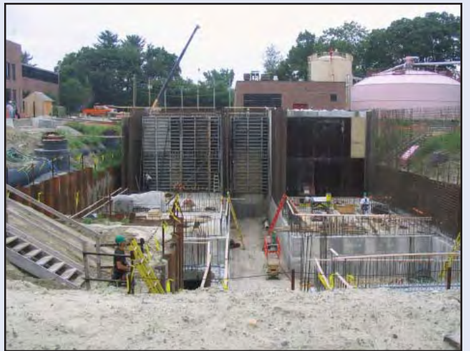
Wet Weather CSO Facility Construction in Nashua, NH.
