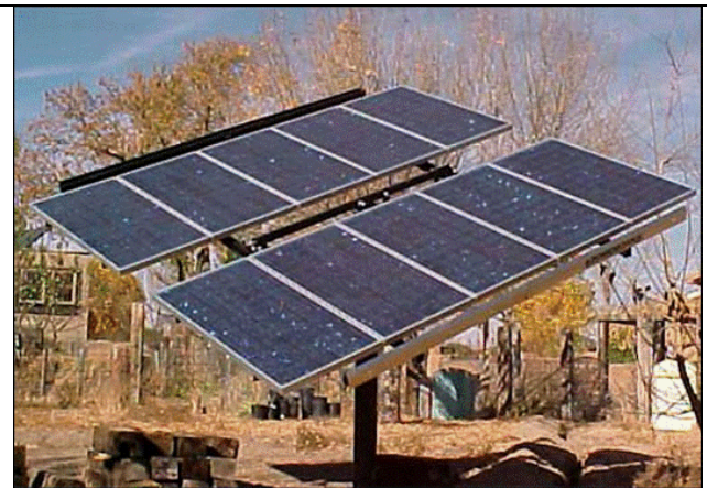
Figure 7 Solar tracking unit. Image courtesy Northern Arizona Wind and Sun 40
