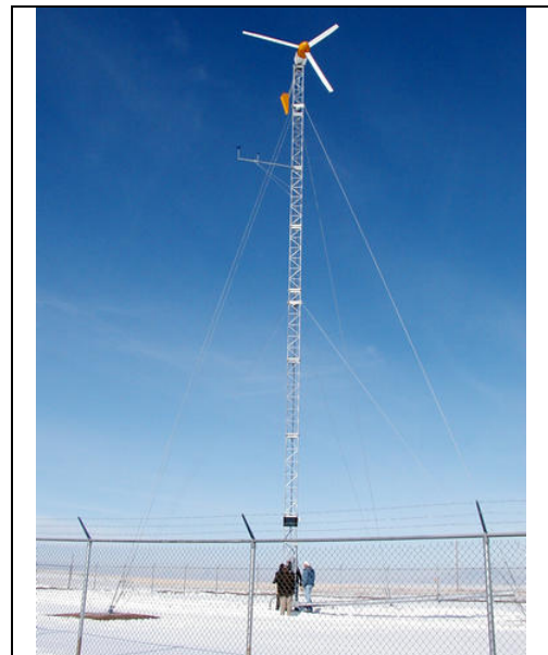
Figure 58 A 10-kW wind turbine with guyed lattice tower. Image courtesy NREL 316
