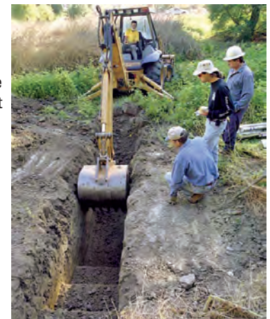
Trenching across the Hayward Fault in Fremont
