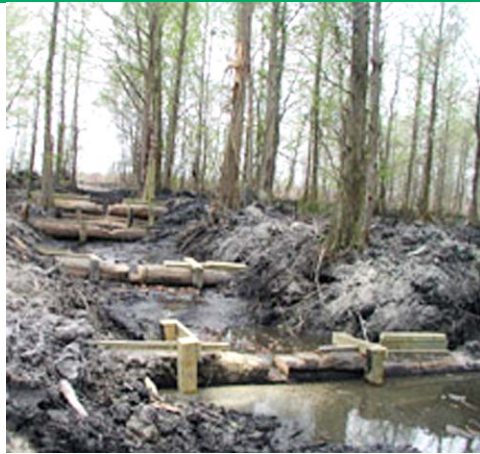
Left: fish ladder under construction; above: a close-up of the construction that helps hold the timber in place.
