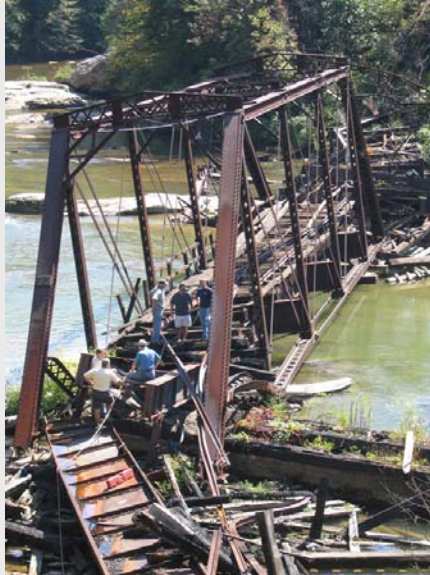
Removal of the collapsed railroad trestle across the Toe River.
